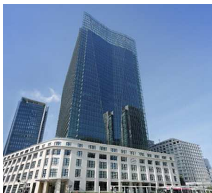
JP TOWER Hall & Conference
